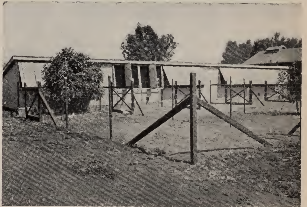
Fig. 66. Poultry yards with removable 8-foot panels in each line fence near the house. End and corner posts are 4 \times 4 inches, line posts are 2 \times 2 inches. Outside line posts require heavier bracing than do the inside posts to allow stretching of extra-heavy fencing around outside.
